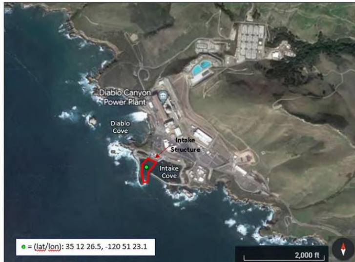
Figure 1-1. Map of the proposed DCPD dredge area (dredge footprint) is outlined in red. Other mapped features include the location of the Intake Structure, the Intake Cove, Diablo Cove, and the DCPD. The approximate geographic center of dredge footprint is the green dot. Latitude (lat) and longitude (lon) for the green dot are shown as degrees, minutes, and decimal-seconds. Image ©2022 Google.
